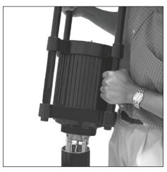
**4.** Install fixture assembly to pole. Orient fixture relative to mount to provide desired lighting distribution.
