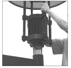
Install fixture assembly on round fitter. Orient fixture relative to mount to provide desired lighting distribution. Tighten securely using 9/16" socket and ratchet with a minimum 12" extension.
