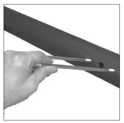
1. Place backing plate inside pole and thread long threaded end of studs into backing plate.
