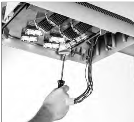
10. Attach EmitterDeck to housing with (4) Phillips screws that were on the original reflector assembly.
