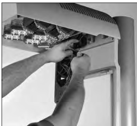
13. Connect disconnect plugs from EmitterDeck to Driver tray. Connect disconnect plugs to power and driver.
