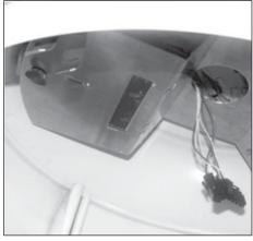
**3.** Separate the disconnect plug halves between the socket & the electronic driver.
