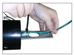
3. Lay pole horizontal on padded supports to protect finish. Pull field wires through pole and out the top. Tie-wrap wires to pole backing plate. Tie field wires in a knot or back loop through tie-wrap. Wire leads need to extend 12" beyond the pole top.
