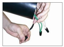
8. Connect field wire leads to fixture leads observing polarity, i.e., green-to-ground, white-to-common, and black-to-voltage.
