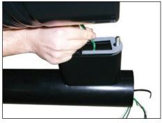
**6.** Insert fixture wire leads through wireway hole while lowering and attaching fixture onto support arm. Pull fixture wire leads out of pole top.
