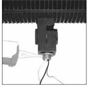
Coat swivel threads with thread sealant to keep moisture from entering junction box.
