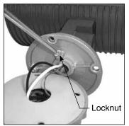
Attach fixture to junction box and orient correctly. Tighten locknut to insure selected orientation.
