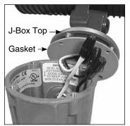
Attach fixture ground lead to circuit ground. Attach fixture leads to circuit leads observing polarity, i.e. whiteto-common and blackto-voltage.
