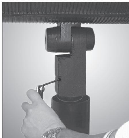
2. Install fixture on tenon, orient, and tighten (2) set screws.
