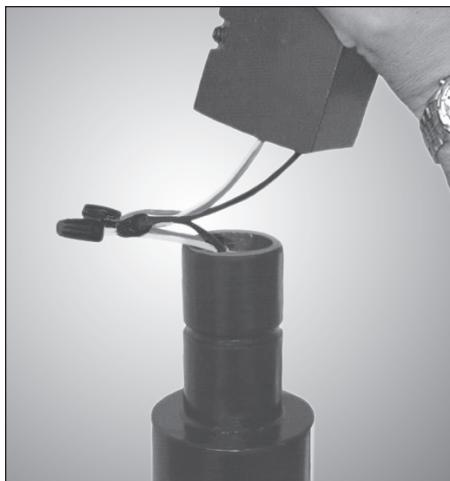
1. Attach fixture leads to circuit leads, observing polarity; i.e.; green-to-ground, white-to-common, and black-to-voltage.
