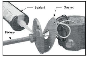
1. Install fixture, coating exposed threads with sealant to keep moisture from entering junction box.
