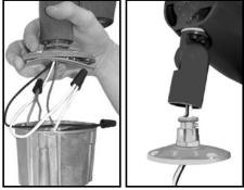
3. Install fixture onto coupling. Attach fixture leads observing polarity, i.e.; green-to-ground, white-to-common, and black-to-voltage.
