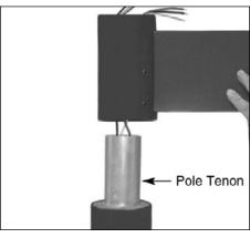
**5.** Carefully slide the slip- fitter over the tenon making sure wires are not pinched.
