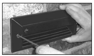
4. Install face plate/gasket assembly and secure with screws.
