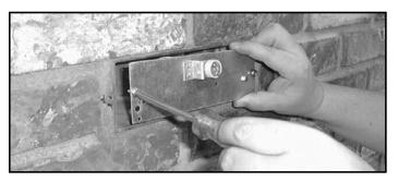
2. Attach fixture wires to field wires using U.L. approved wire nuts ensuring correct polarity, i.e., green-to-ground white-to-common, black-to-voltage. Install ballast / socket plate and tighten screws securely. Install lamp of type and wattage as shown on fixture label and chart on this page (not needed for L.E.D. fixture).
