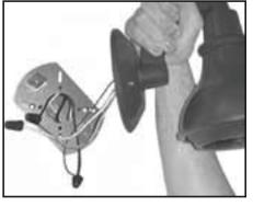
Attach fixture leads to circuit leads observing polarity, i.e. green-toground, white-to-common, and black-to-voltage. Push wire connections back into j-box.
