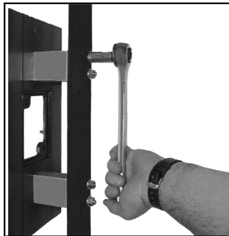
11. Install crook arm onto bolts and secure with washers and nuts. Tighten to 20 ft.-lbs.
