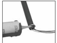
2. Coat threads with a good sealant and install pole into desired junction box. (Direct burial box for H.I.D.)
