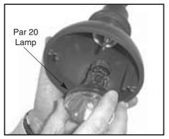
Install lamp of type and wattage shown on fixture label & chart.
