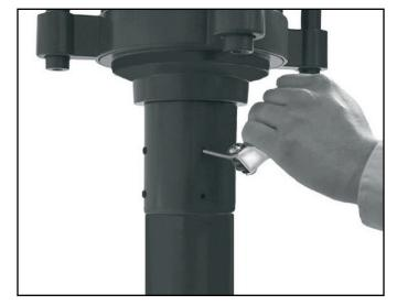
3. Tighten (4) set screws securely using a <sup>3</sup>/<sub>16</sub>" hex wrench. Remove one screw, drill recess in tenon or pole for screw point, and replace set screw.
