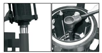
6. Install fixture onto round fitter. Orient fixture relative to mount to provide desired lighting distribution. Tighten securely using %16" socket, extension and ratchet.
