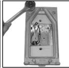
Apply a continuous bead of sealant compound into the wall plate groove. Allow mastic to extend well above the wall plate surface to ensure a proper seal. Securely mount wall plate over junction box on wall (hardware provided by others).
