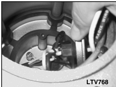
8b. Make wire connections observing polarity, i.e.; green-to-ground, white-to-common, and black-to-voltage. Replace splice compartment cover. Tighten cover screws to 15 inch/pounds, (1¼ ft. lbs.)
