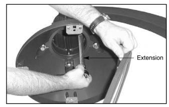
4. Using long socket extension, tighten to 20 ft.-lbs. IMPORTANT NOTE! ORIENT "HINGE" SIDE OF FIXTURE TOWARDS POLE.
