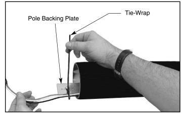
3. Lay pole horizontal on padded supports to protect finish. Pull wires through pole & out the top. Tie-wrap wires to pole backing plate. Tie wires in a knot or back loop through tie-wrap. Wire leads need to extend 12" beyond the hand hole.
