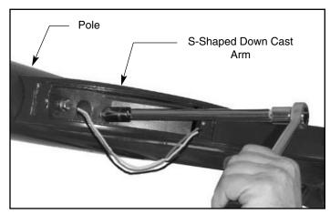
4. Attach down cast arm to pole. Tighten to 20 ft.-lbs.
