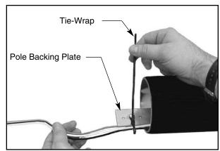
2. Lay pole horizontal on padded supports to protect finish. Pull wires through fixture base, arm, into pole wireway hole & out the pole top. Tie-wrap wires to pole backing plate. Tie wires in a knot or back loop through tie-wrap. Wire leads need to extend 12" beyond the pole top.
