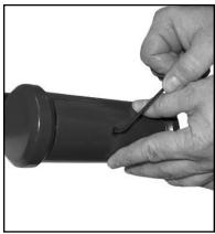
Attach fitter cover using a hex wrench. Make wire connections at pole hand hole observing polarity, i.e.; green-to-ground, white-tocommon and black-tovoltage.
