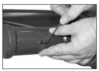
Attach fitter cover using a hex wrench. Make wire connections at pole hand hole, observing polarity, i.e.; green-to-ground, white-to-common and black-to-common.
