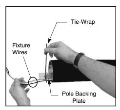
3. Lay pole horizontal on padded supports to protect finish. Pull field wires through pole & out the top. Tie-wrap wires to pole backing plate. Tie field wires in a knot or back loop through tie-wrap. Wire leads need to extend 12" beyond the pole top.
