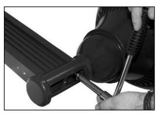
5. Attach ribbon arm loosely to pole by sliding arm over rods and making sure wires are pulled tight so they do not get pinched. Connect fixture wires to field wires observing polarity, i.e.; greento-ground, white-to- common, and black-tovoltage. (See fixture installation instructions.)
