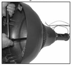
Attach fixture head to arm fitter using a torque wrench. Pull wires making sure they do not get pinched.
