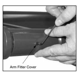
7. Install arm fitter cover. Make wire connections at pole hand hole, observing polarity, i.e; green-to-ground, white-to-common and black-to-voltage.
