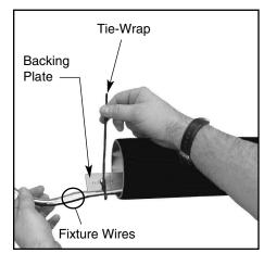
3. Lay pole horizontal on padded supports to protect finish. Pull wires through pole & out the top. Tiewrap wires to pole backing plate. Tie wires in a knot or back loop through tie-wrap. Wire leads need to extend 12" beyond the pole hand hole.
