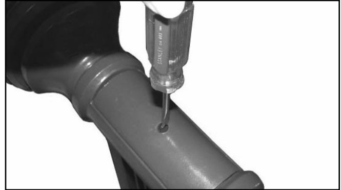
6. Install arm fitter cover. Make wire connections at pole hand hole observing polarity, i.e.; green-to-ground, white-to-common and black-to-voltage.
