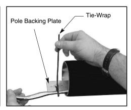
2. Lay pole horizontal on padded supports to protect finish. Pull wires through fixture base, arm into pole wireway hole & out the top. Tie-wrap wires to pole backing plate. Tie field wires in a knot or back loop through tie-wrap. Wire leads need to extend 12" beyond the pole top.
