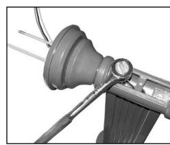
Install arm fitter assembly to ribbon arm. Connect fixture wires to field wires at pole hand hole observing polarity, i.e.; green-to-ground, whiteto-common, and black-to-voltage.
