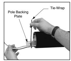
3. Lay pole horizontal on padded supports to protect finish. Pull field wires through pole & out the top. Tie-wrap wires to pole backing plate. Tie wires in a knot or back loop through tie-wrap. Wire leads need to extend 12" beyond the pole top.
