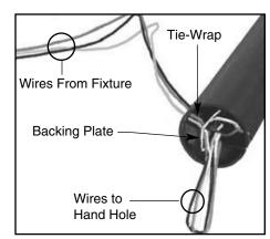
3. Lay pole horizontal on padded supports to protect finish. Pull wires through pole & out the top. Tie-wrap wires to pole backing plate. Tie wires in a knot or back loop through tie-wrap. Wire leads need to extend 12" beyond hand hole.
