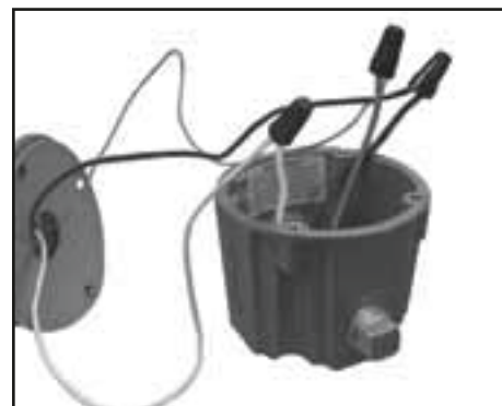
3. Attach fixture leads observing polarity; i.e.; braided bare copper wire-to-ground, white-to-common, and black-to-voltage.
