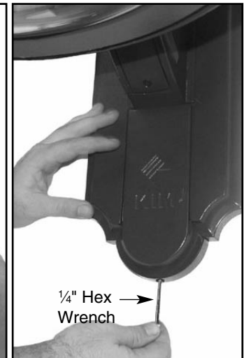
7. Attach splice cover using the 10-32 flat head socket stainless steel screw.
