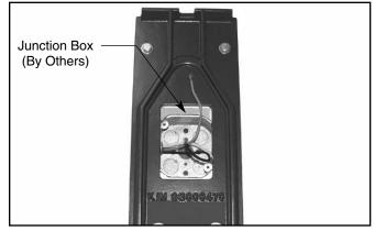
Securely mount wall plate over junction box (by others) on wall. CAUTION: Structural integrity of mounting plate attachment to wall is by others.
