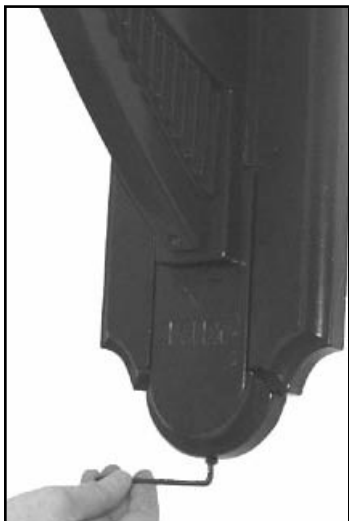
8. Attach splice cover using the 10-32 flat head socket stainless steel screw.
