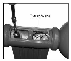
Pull fixture wires through arm fitter, ribbon arm and wall plate cover. Install arm fitter with fixture head to ribbon arm using a torque wrench.
