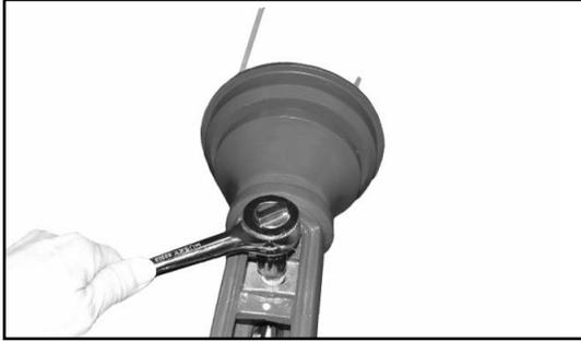
6. Feed fixture wires from arm fitter through ribbon arm. Install arm fitter assembly to ribbon arm using torque wrench. (See fixture installation instructions for fixture attachment.)
