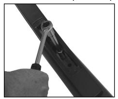
1. Install side pole swept cast arm hub to pole with bolts, tighten to 20 ft.-lbs. All mounting hardware is supplied by Kim Lighting.
