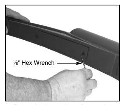
Push wire into pole and out pole hand hole. Secure wire with the cable tie provided. Install arm access cover and secure with screws.
