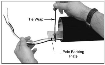
Lay pole horizontal on padded supports to protect finish. Pull wires through pole & out the top. Tiewrap wires to pole backing plate. Tie wires in a knot or back loop through tie-wrap. Wire leads need to extend 12" beyond the handhole.
