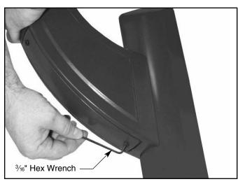
5. Push wires into pole and out pole handhole. Secure wire with the cable tie provided. Install arm access cover and secure with screws.
