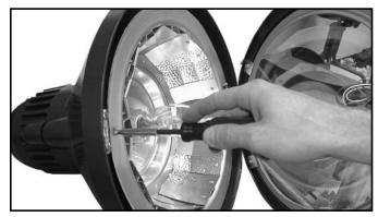
6. Secure reflector with ¼ turn fastener. Install lamp of type and wattage shown on fixture label, close and secure fixture door.
