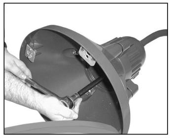
2. Install fixture head to crook arm with bolts, tighten to 20 ft.-lbs. **NOTE: Orient "hinge" side of fixture towards the pole.**
