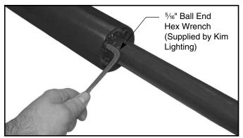
3. Feed wires through pole and out hand hole. Install crook arm to pole with bolts in desired orientation, tighten to 20 ft - lbs.
