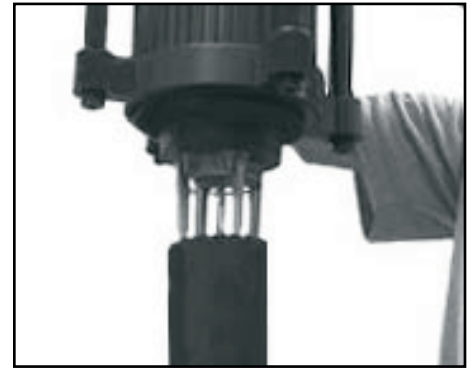
4. Install fixture assembly to pole. Orient fixture relative to mount to provide desired lighting distribution.
