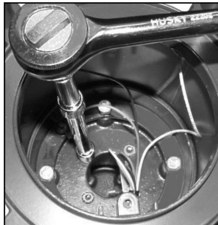
9. Orient fixture relative to mount to provide desired lighting distribution. Secure with washers and nuts using a \frac{9}{16} " ratchet wrench with 10" extension.
