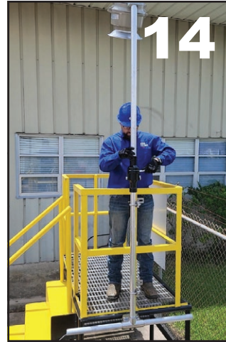
14 TIGHTEN THE HINGE TOP SET SCREWS. TIGHTEN THE LOCK BOLT
