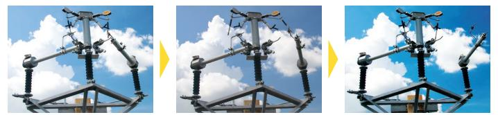
The pick-up finger engages the actuator rod creating a parallel current path. At a pre-determined point, the vacuum contacts separate, interrupting the circuit.
