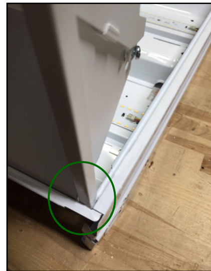
Figure 7. Hinges slid backwards towards side of housing.
