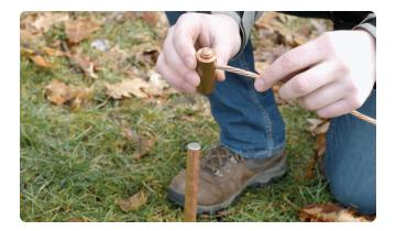
**Step 3 –** Drive the HammerTap onto the ground rod using a hammer.
