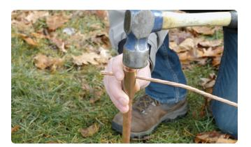
**Step 4 –** Hammer until the nub of the HammerTap is flush with the HammerTap body. Once it is flush, the connection is complete.
