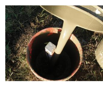
The four main ingredients for Helical Pulldown Micropile grout are Portland type I or II cement, microsil aggregate, and water. Retarders, plasticizers, and expansive agents can be added as necessary.
