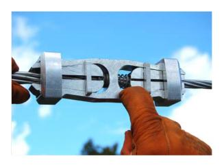
5) Visually confirm that wire is all the way in and the strands are not separated.
