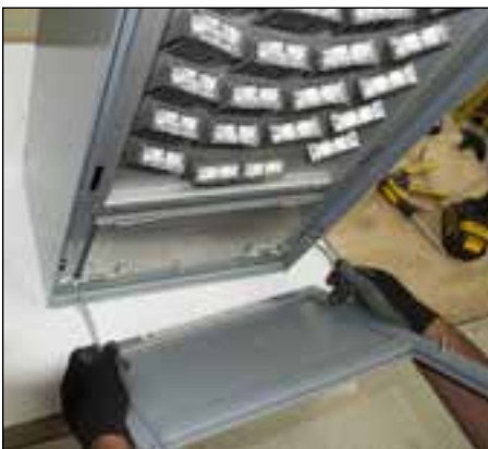
31. Re-hang lens frame into fixture housing.
