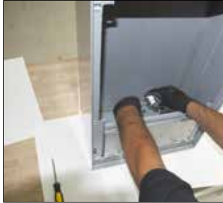
8. Unplug quick-disconnects between reflector assembly and ballast assembly.
