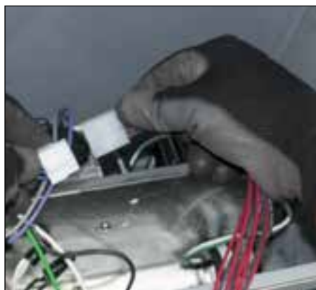
23. Attach quick-disconnects between new PicoPrism™ deck and electronic driver.
