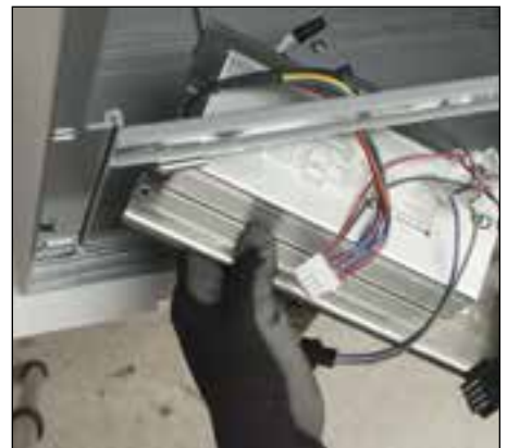
18. Raise new electronic driver tray into driver compartment.
