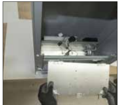
21. Re-attach existing ballast assembly door by sliding it back onto hinges on the housing.
