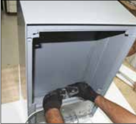
7. Unplug quick-disconnects between ballast assembly and line voltage.
