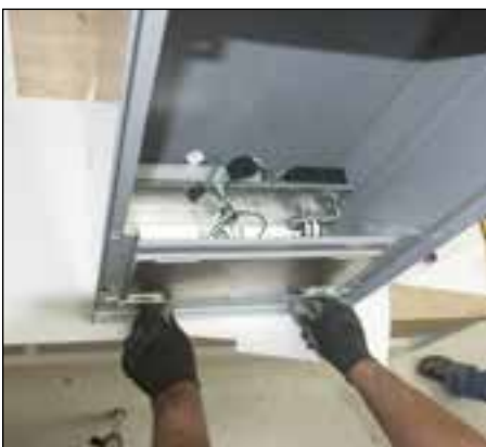
22. Grasp ballast assembly slip hinges and slide inward to lock into place on housing.
