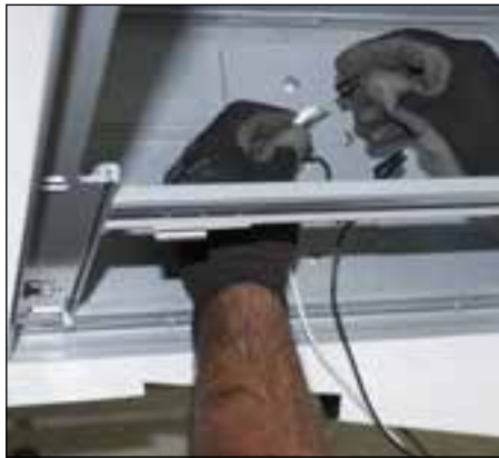
17. Using wire connector by others, attach new harness to line voltage.
