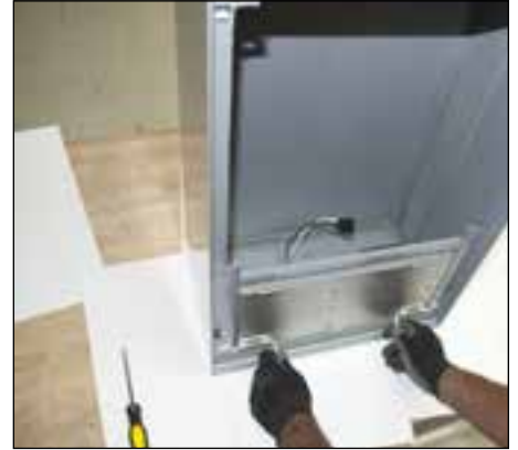
9. Grasp ballast assembly slip hinges and slide inward to open ballast assembly door hinges.
