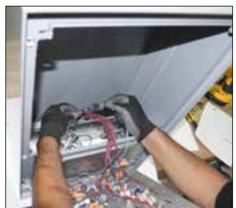
24. Attach quick-disconnects between driver dimming lead and PicoPrism deck.
