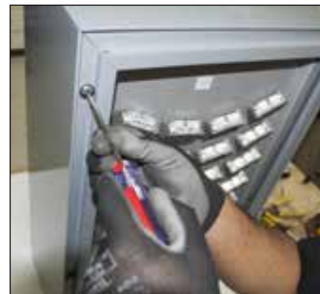
32. Raise lens frame assembly into place and re-attach to housing with four (4) slotted-head fasteners.
