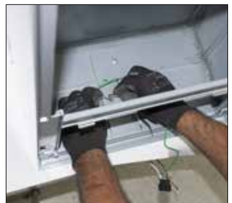
15. Install new grounding wire.
