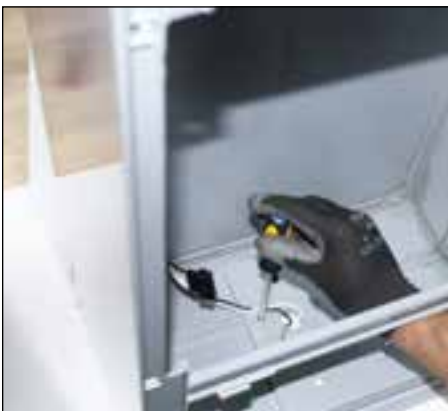
13. Unscrew plastic clamp holding wires from line voltage.
