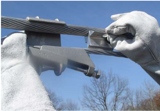
6) Slide interface between conductors and into the connector until it reaches the stop.
