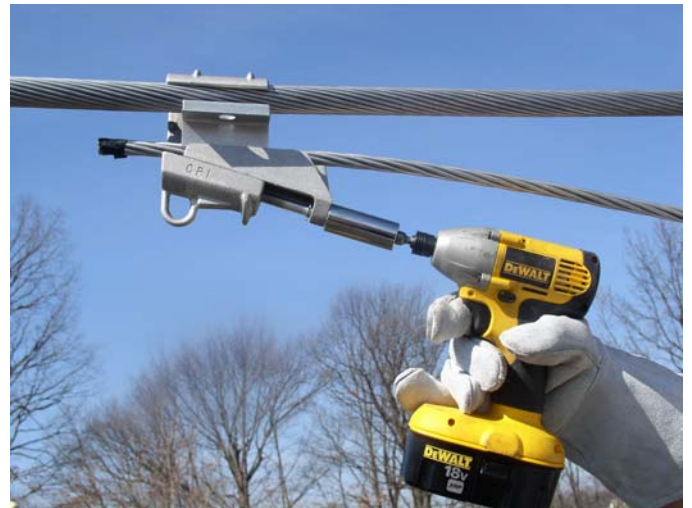
7) Use any 3/4" socket to drive the bolt until the head breaks off. Any impact, box, adjustable, speed or socket ratchet wrenches will work.
