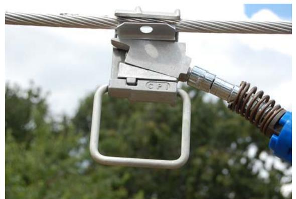
12) Use a universal socket stick and 3/4" socket to tighten bolt until Hex Head shears off. The bolt should break off at 110-130 INLBS (12-14 NM)
