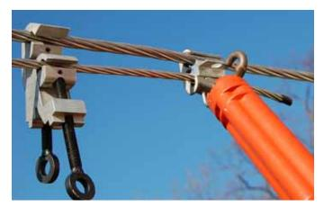
10) Release interface from hot-stick. Make sure it is fully inserted against the stop.
