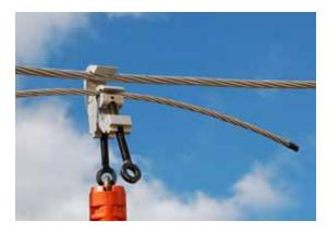
1) Attach TAP wire in PIGGYBACK CLAMP. Leave 10"- 20" (25 cm - 50 cm) of wire exposed.
