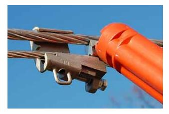
9) Slide INTERFACE along MAIN CONDUCTOR until it reaches the stop.
