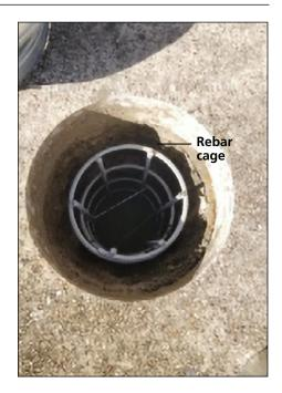
2. Center the rebar cage provided in the hole excavated. Be sure that the rebar cage is oriented correctly in the hole. The top of the rebar cage has a ring welded approximately flush with the top of the vertical bars. Gravel can be used to adjust the rebar cage height during positioning.
