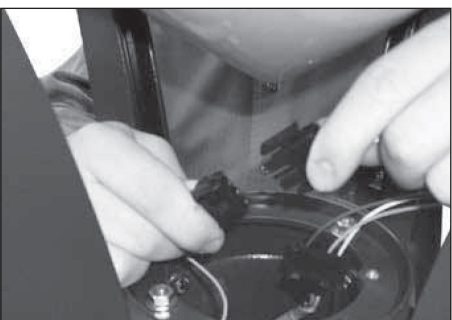
22. Connect supplied harness to pole wiring and the fixture wiring quick disconnects.
