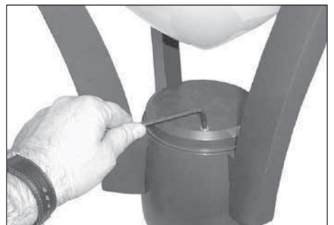
12. Remove wiring access cover from fixture hub.
