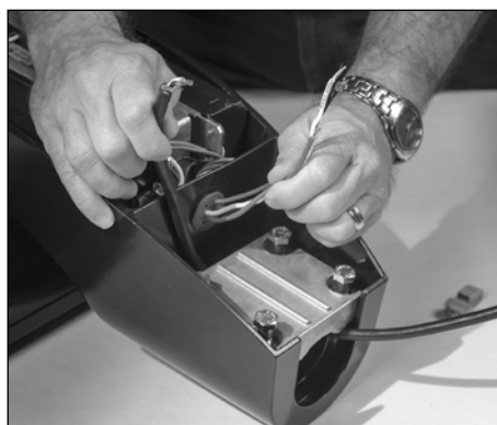
5. Pull wiring from line voltage over the top of the tenon clamp.
