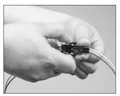
**10.** Connect quick-disconnects from fixture head to driver.
