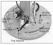
4. Install the base casting/driver assembly on the pre-set anchor bolts. Use flat washer and hex nuts both below and above the casting.
