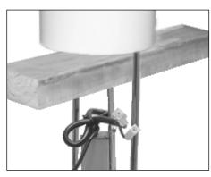
**8.** Place wooden block, (by others), on top of driver assembly for easier wiring.
